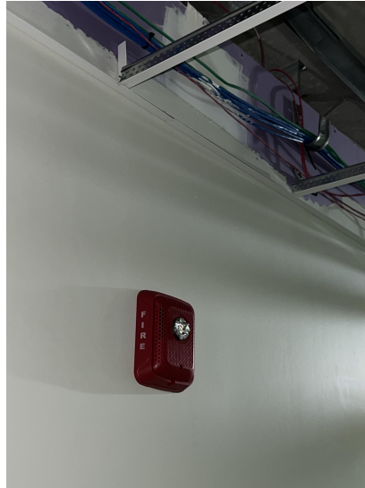
Installing fire alarms throughout level 2.
